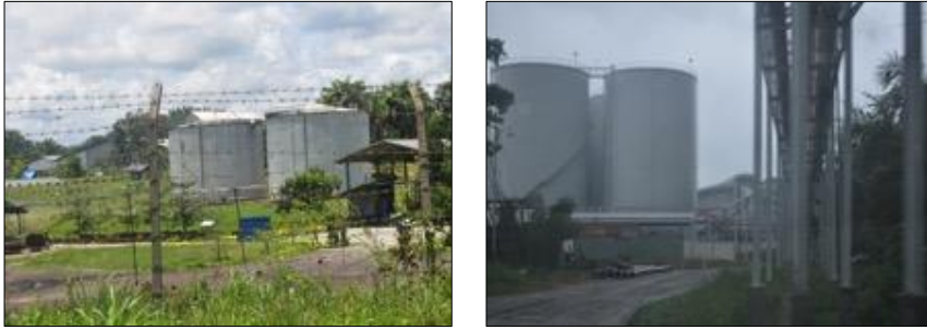
Figure 4. KPO and CPO storage tanks in the mills in North Mamuju
