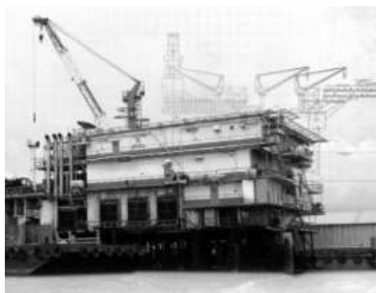
Gambar 2. Offshore Rig PT. Apexindo Pratama Duta Tbk
