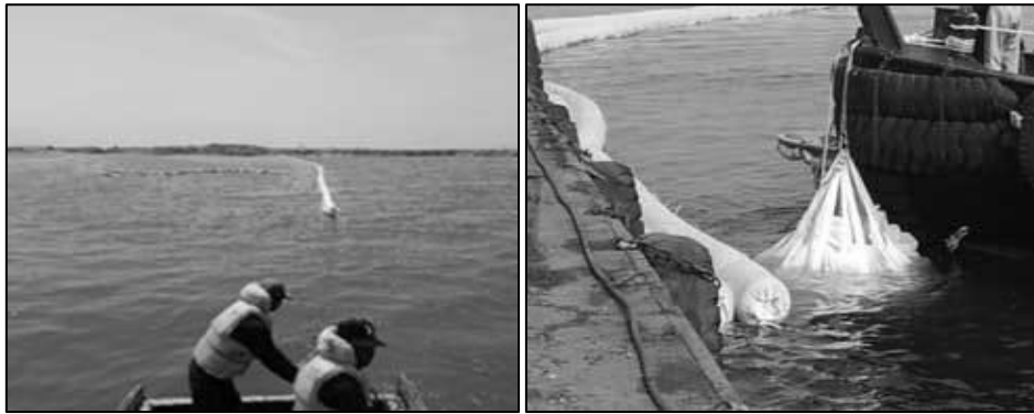
Gambar 3 Proses Instalasi Silt Curtain
