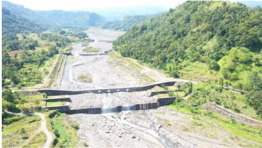
Image 3. The sand pocket in middle-stream area of Jeneberang River (Source: Author provided)
