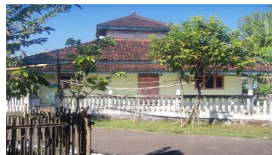
Figure 15. The condition of the village road was moved about 50 m from the beach.
