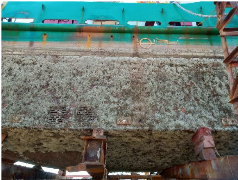
Figure 1. Corrosion on Ship Plates
