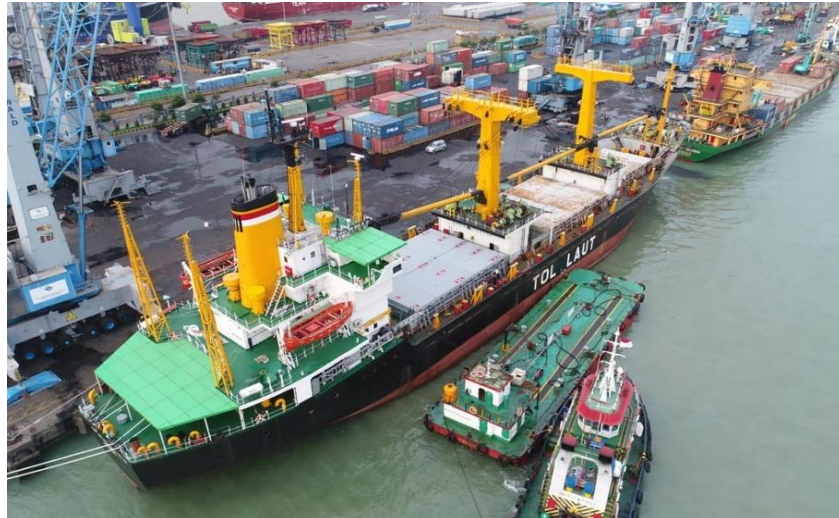
Figure 1. Tanjung Surabaya Container Port Pier
