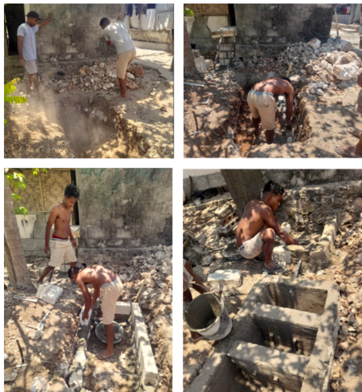
Gambar 5. Pelaksanaan instalasi water treatment
