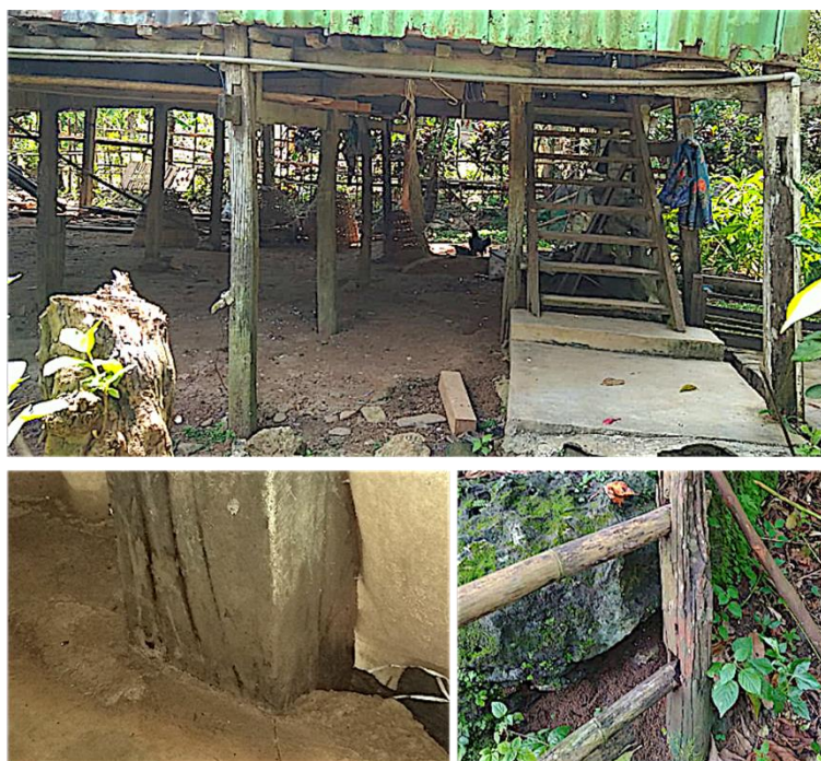
Figure 4. Wood of H. celebica installed directly into the ground without needing to be supported using footing
