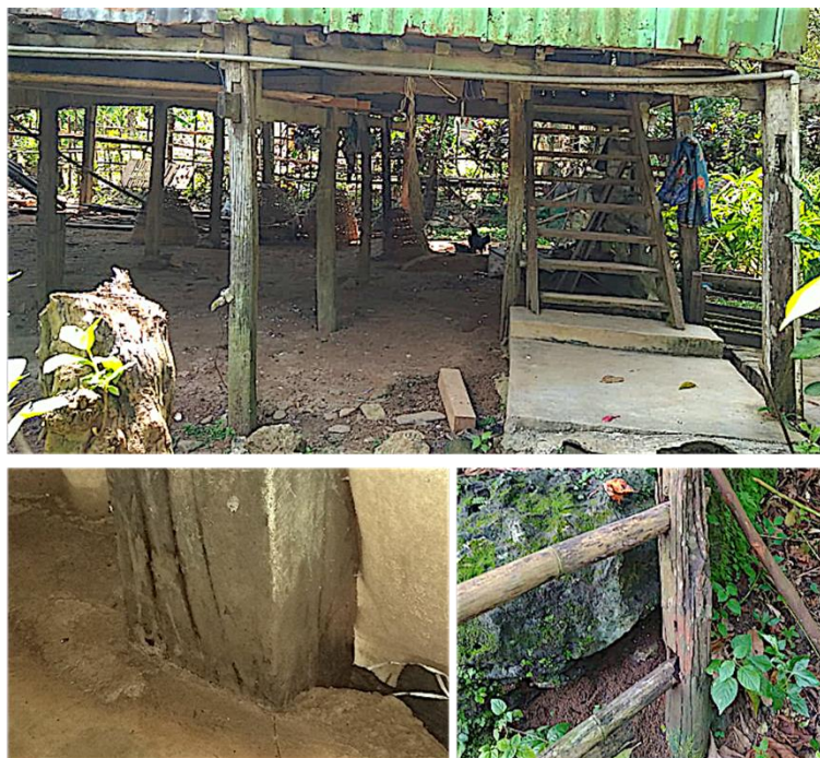
Figure 4. Wood of H. celebica installed directly into the ground without needing to be supported using footing
