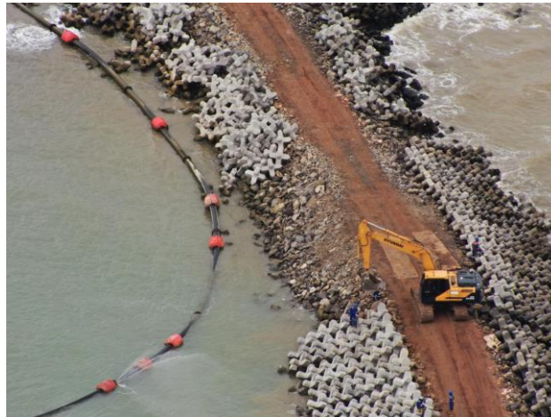
Figure 9. Installation on the West Groin [13]
