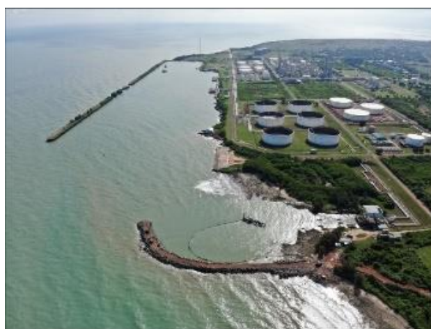
Figure 7. Location of Groin Structure [12]
