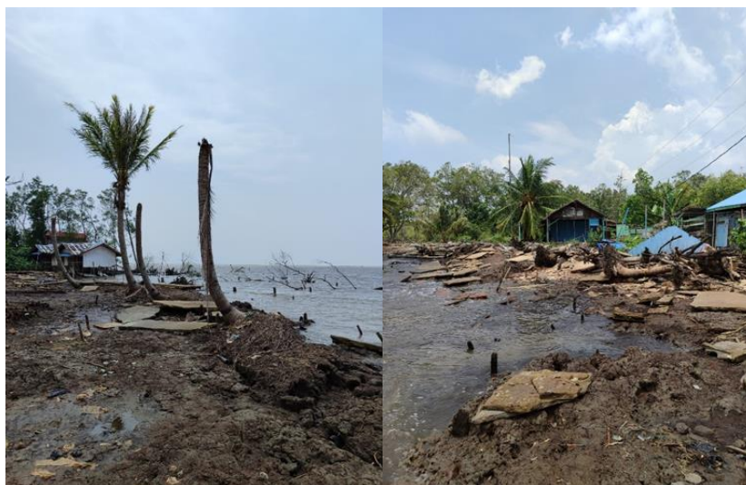
Figure 6. Documentation of abrasion in the Kuala Karang Village area
