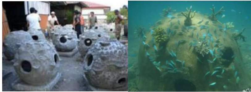
(a) Construction of reef balls; (b) Condition of reef balls after several years of use Figure 5. Reef ball type artificial reef in Karang Jeruk waters [13]
