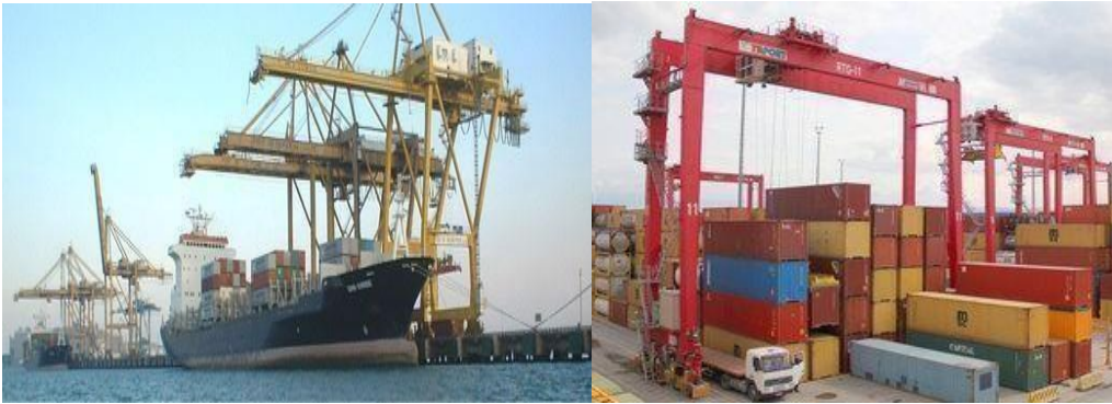
Figure 1. Condition of the New Makassar Container Terminal, 2024.
